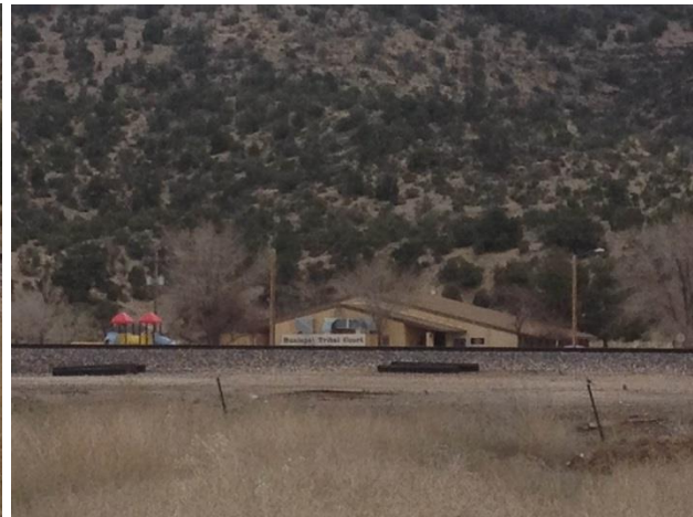
Image 4. Overpass #3 Court House (North)
