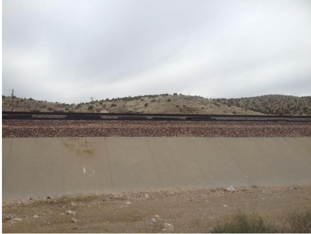
Image 5. Overpass #4 Park (South)
