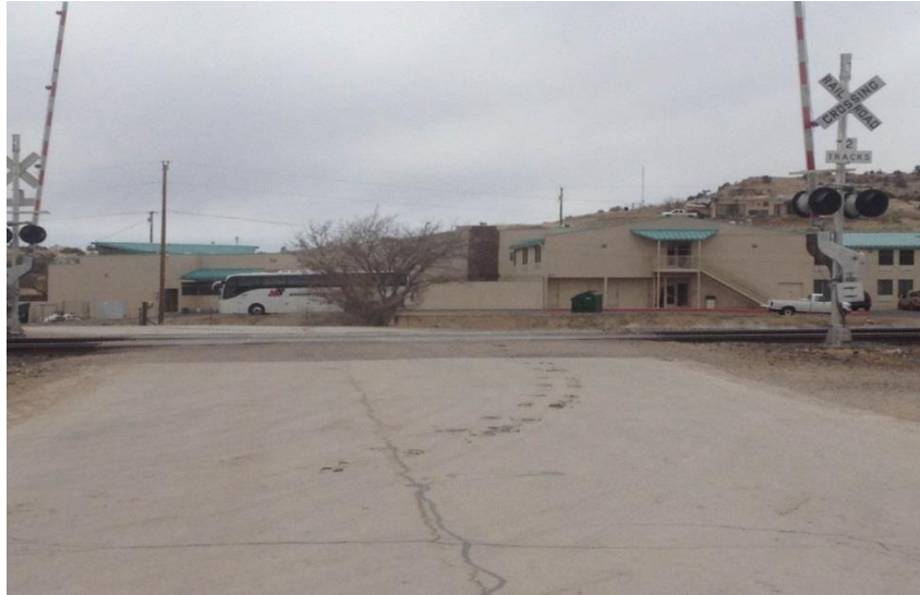
Image 1. At-Grade Crossing In Peach Springs
