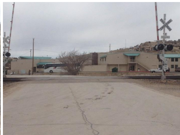
Image 8. Overpass #2 Main Road (North)
