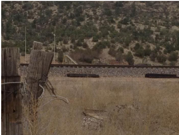
Image 3. Overpass #4 Park (North)
